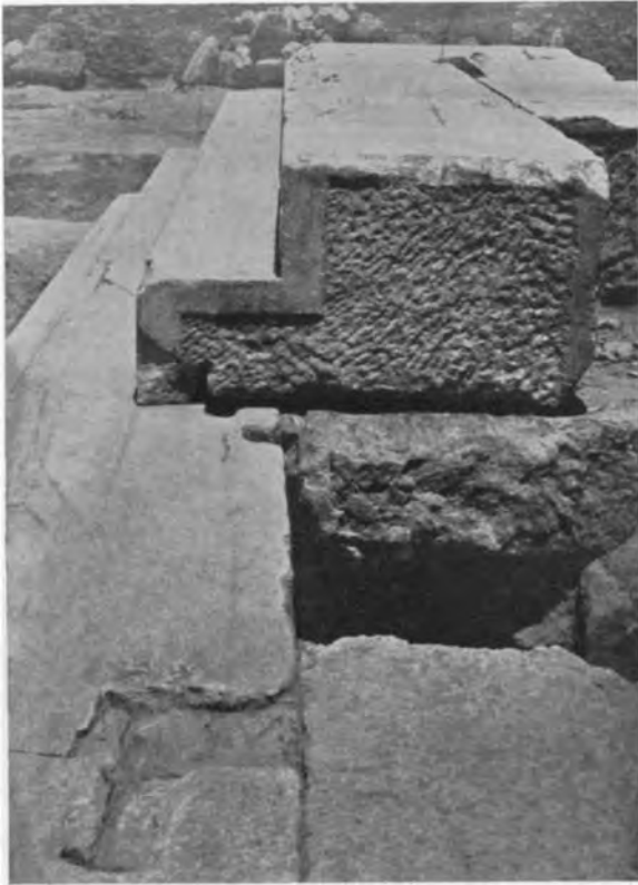
Fig. 28. Detail of Holes for Clamps and Dowels
