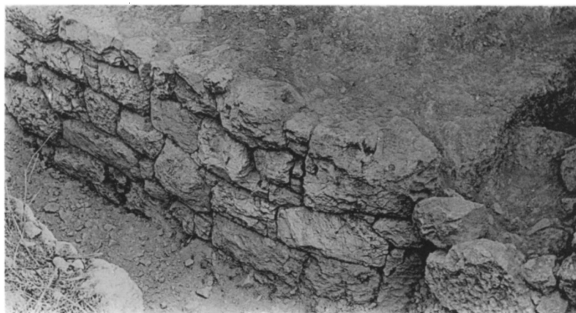
d. E. Wall of Drain at Entrance of Side-Drain. Crude Dam across Mouth of Side-Drain at right
