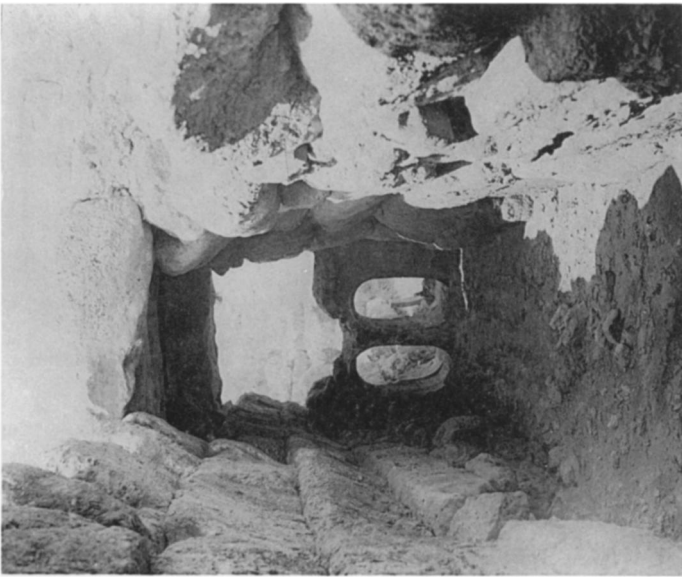
a. Great Drain, looking N. at Bridge: Corbelled W. Wall (left)
