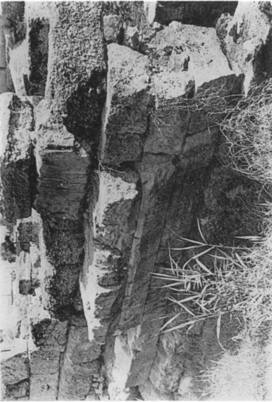
b. Corbelled Construction beside the Eridanos at the Kerameikos
