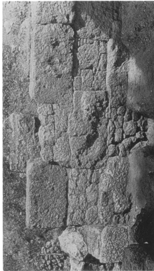
e. W. Wall of Drain = E. Wall of House A, Second Period: "Checkerboard" Construction
