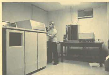
Sarah George Figueira, In-House Production Manager, removes from the typesetter the cassette containing the typeset pages for development on the processor. In the background: the tape drive (left) and central processing unit (right)
