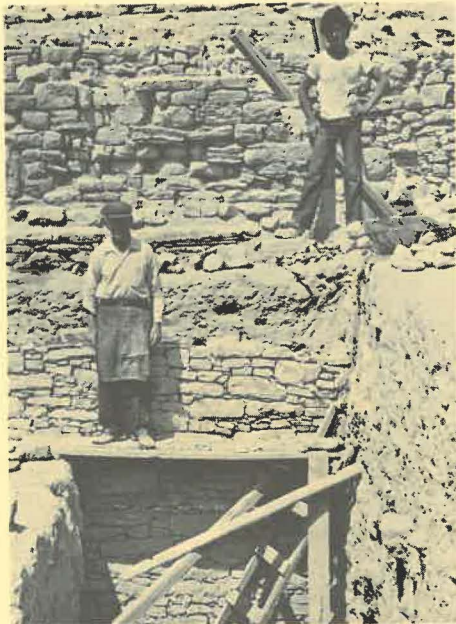
A supporting wall to protect against erosion is constructed at Kommos. The section reveals walls of the Hellenistic court built on top of the earlier wall. The Hellenistic walls begin at the shoulder level of Aristotle, the 78 year old mason standing at center. Above right in the Hellenistic court is his grandson, Antonis
