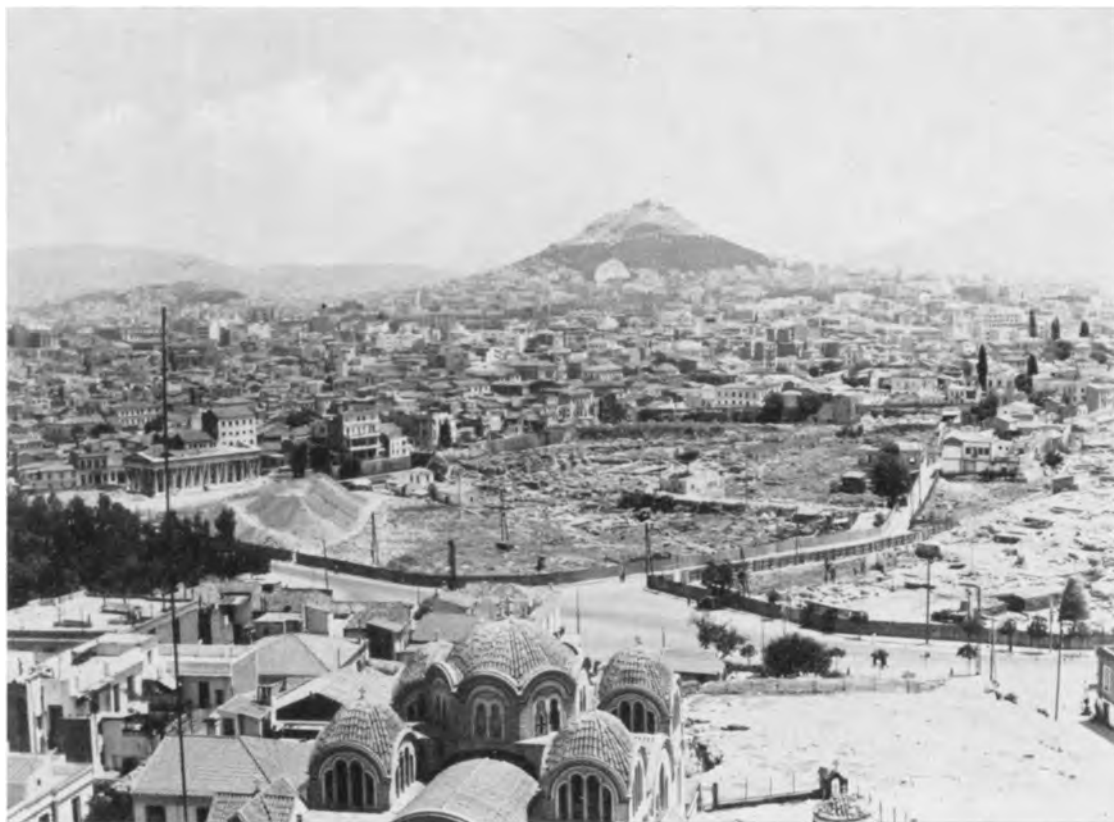
Fig. 1. Northern Part of the Excavated Area
