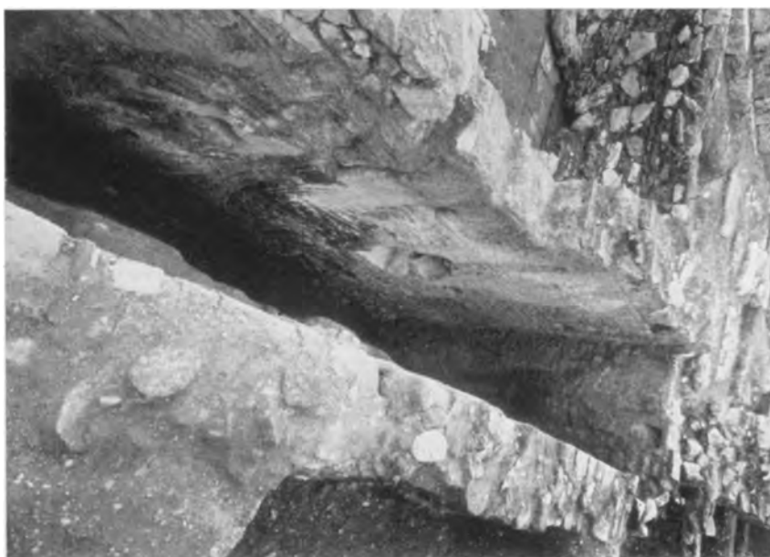
Fig. 3. East and South Walls of Wheel-race, from North
