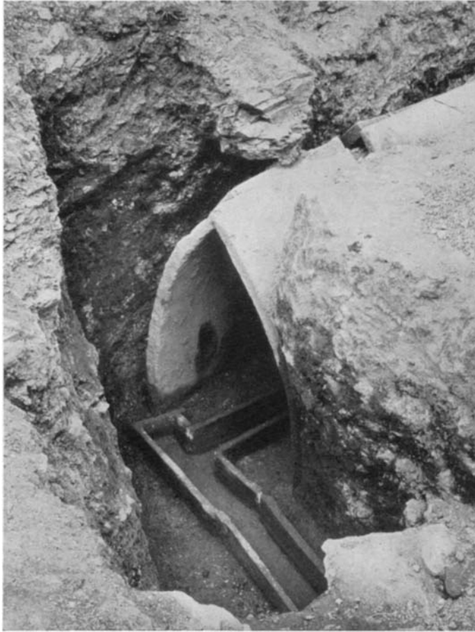
Fig. 4. Corner of Water-channel
