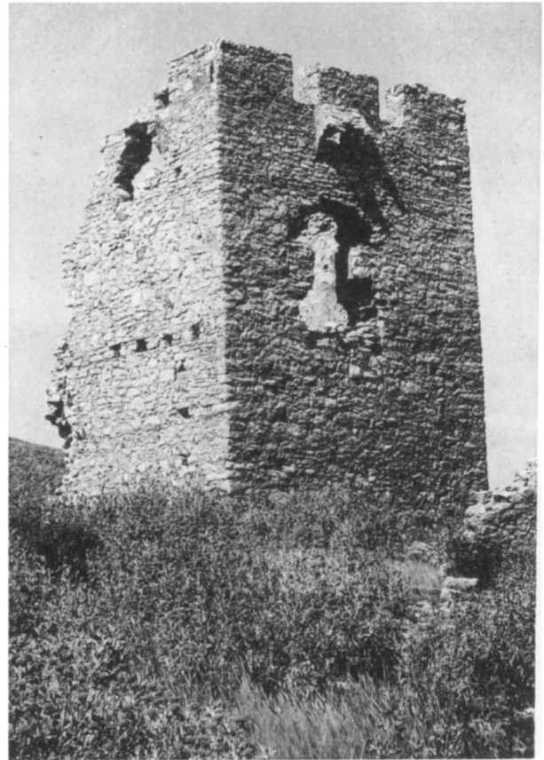
b. Tower of the Princess, from Southwest.
