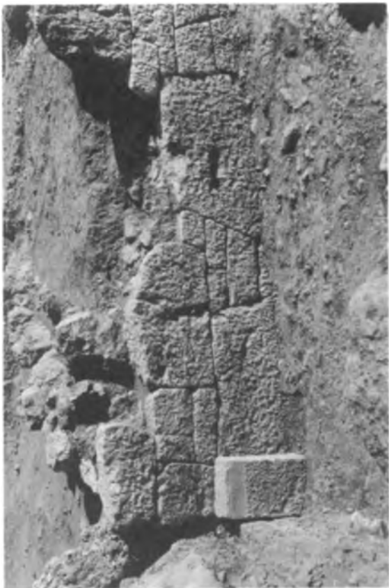
b. Outer Face of Northwest Wall with Boundary Stone
