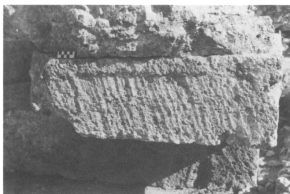
e. Temple of Apollo (6th century), foundation of north colonnade from the west
