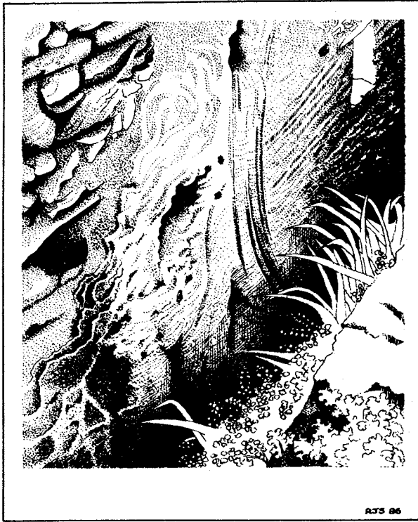
FIG. 1. Lime deposits on the east wall of the water-wheel pit
