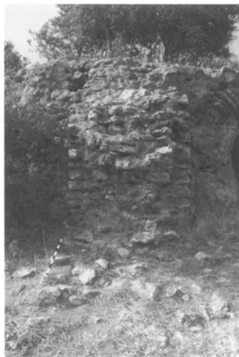
b. Bulky middle buttress of curved opus arcuatum at Belanidia, from south
