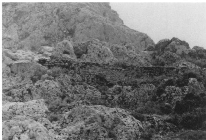
b. Supporting wall of aqueduct at Agios Basileios, from north
