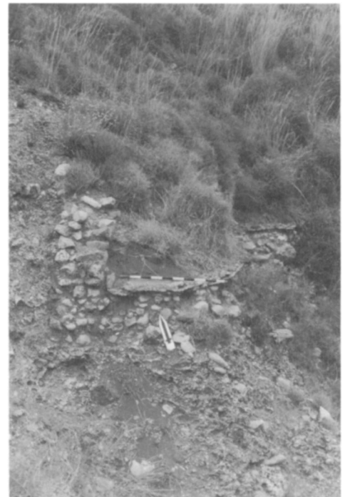
c. Anaploga: conduit on western flank of ravine, from south
