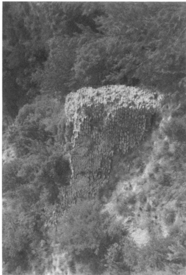
a. North wall of bridge of Skouroukli, from west
