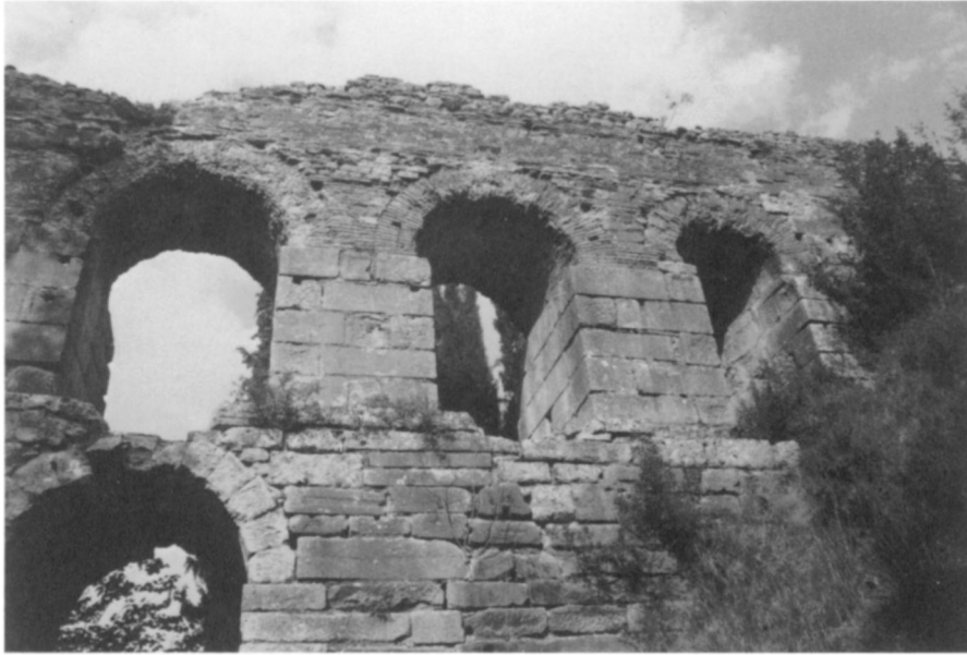
a. Bridge at Stroggylo, north face
