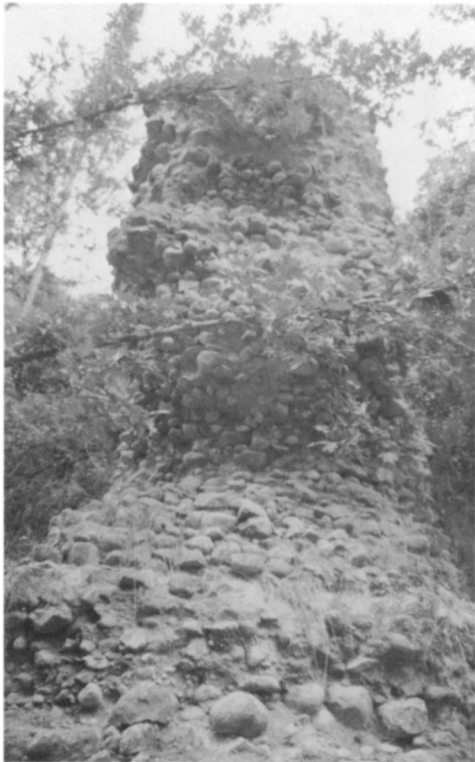
c. Eastern pier of bridge at Kabourorema
