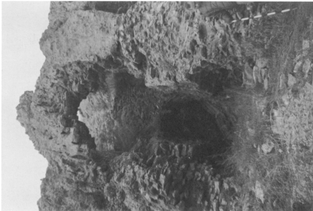
a. Ntourmiza: inner, lower arch and two buttresses of supporting wall, from north
