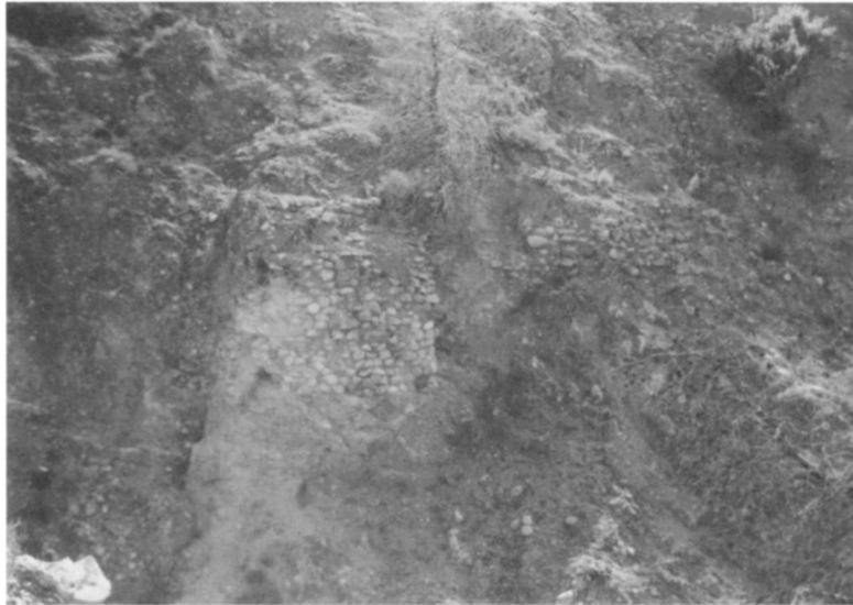
a. Aqueduct on slope of Kastraki, from west
