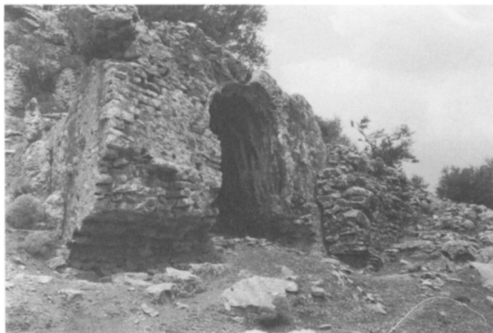
a. Easternmost arch at Belanidia reinforced by wall, from southwest
