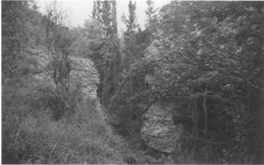
a. Piers of bridge at Kabourorema, from south
