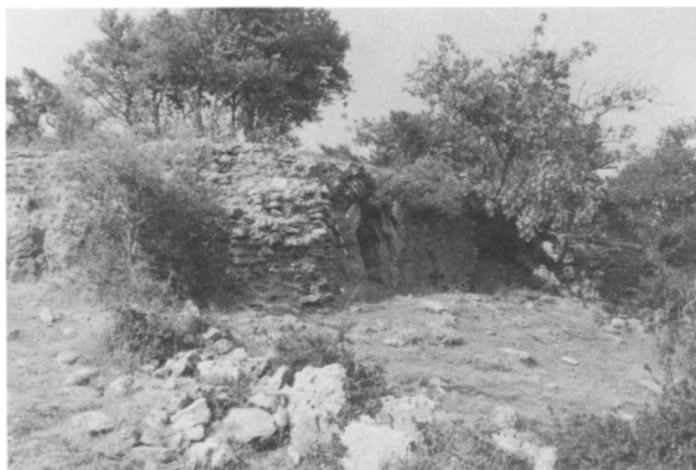
e. Belandia: bulky buttress in middle of supporting wall, from south
