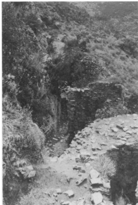
a. Top of arches at Ntourmiza, from east
